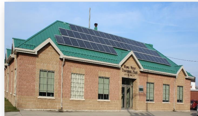
Water Treatment Plant Wawa, ON
